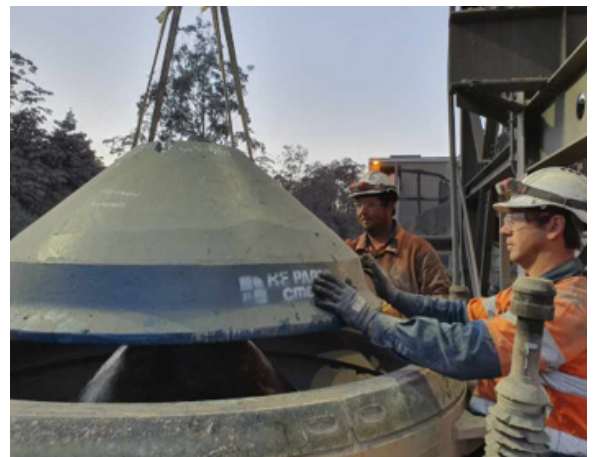
Optimized CME™ MnElite liners being installed
